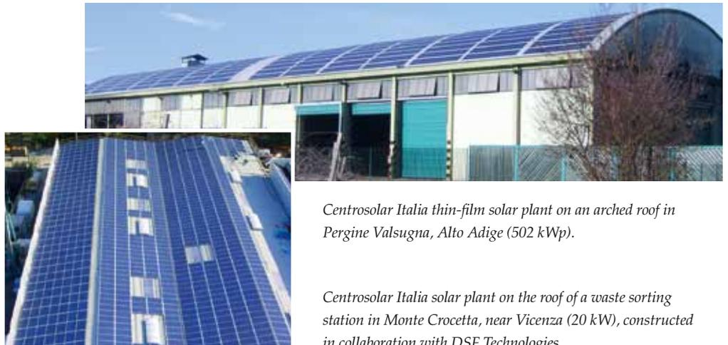
*Centrosolar Italia thin-film solar plant on an arched roof in Pergine Valsugna, Alto Adige (502 kWp).*
